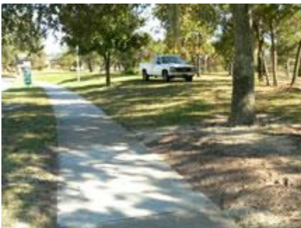
Sidewalk after root excavation
