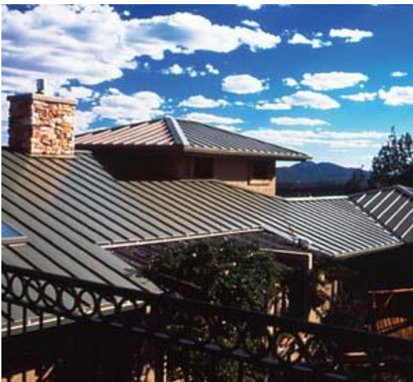
Figure 5- This is an example of a “cool roof,” which is made from materials that force solar heat away from the building.
